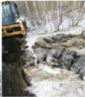
Photo 18 Trench burial needs the use of an excavator
