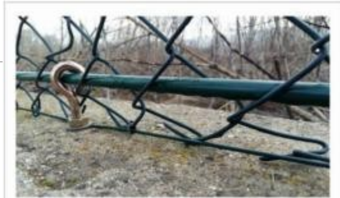
Figure 2.5. Anchoring a mesh to a wall with a horizontal metal rod to prevent mesh lift
