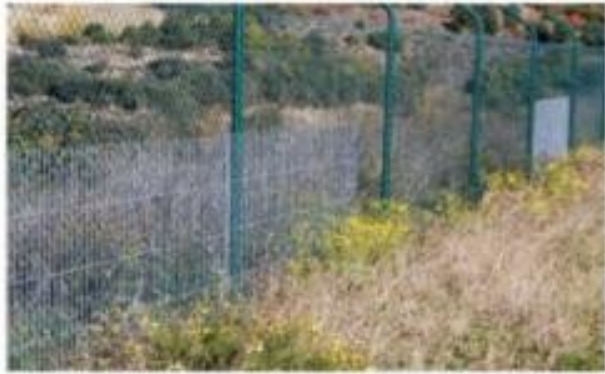
Figure 2.1. Fence reinforced with electro-welded mesh
