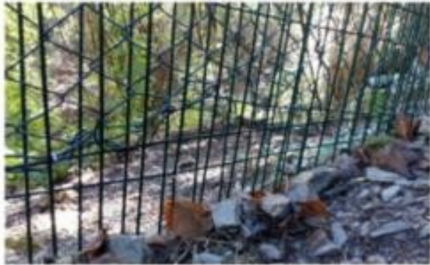
Figure 2.3. Damaged torsion mesh reinforced with an electro-welded mesh.
